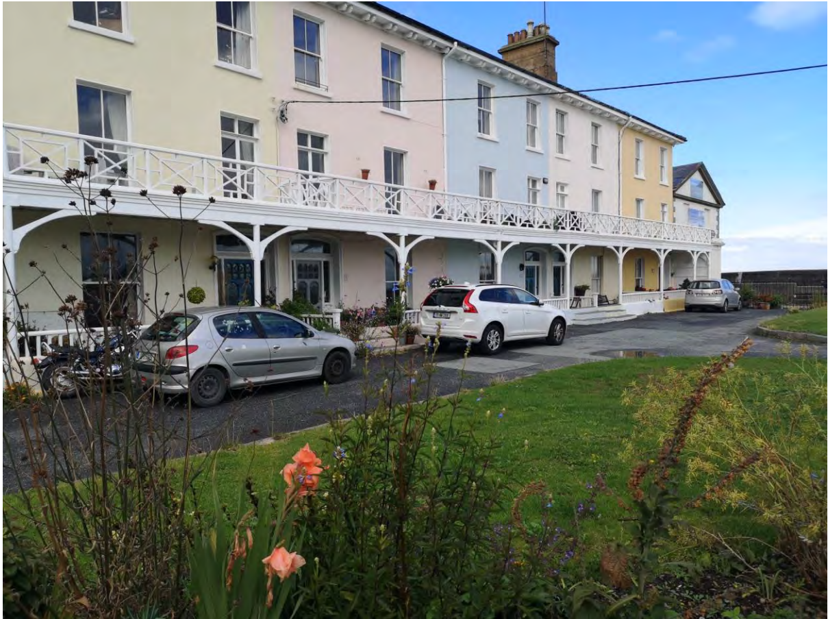
Figure 3.8: Martello Terrace, Strand Road.
