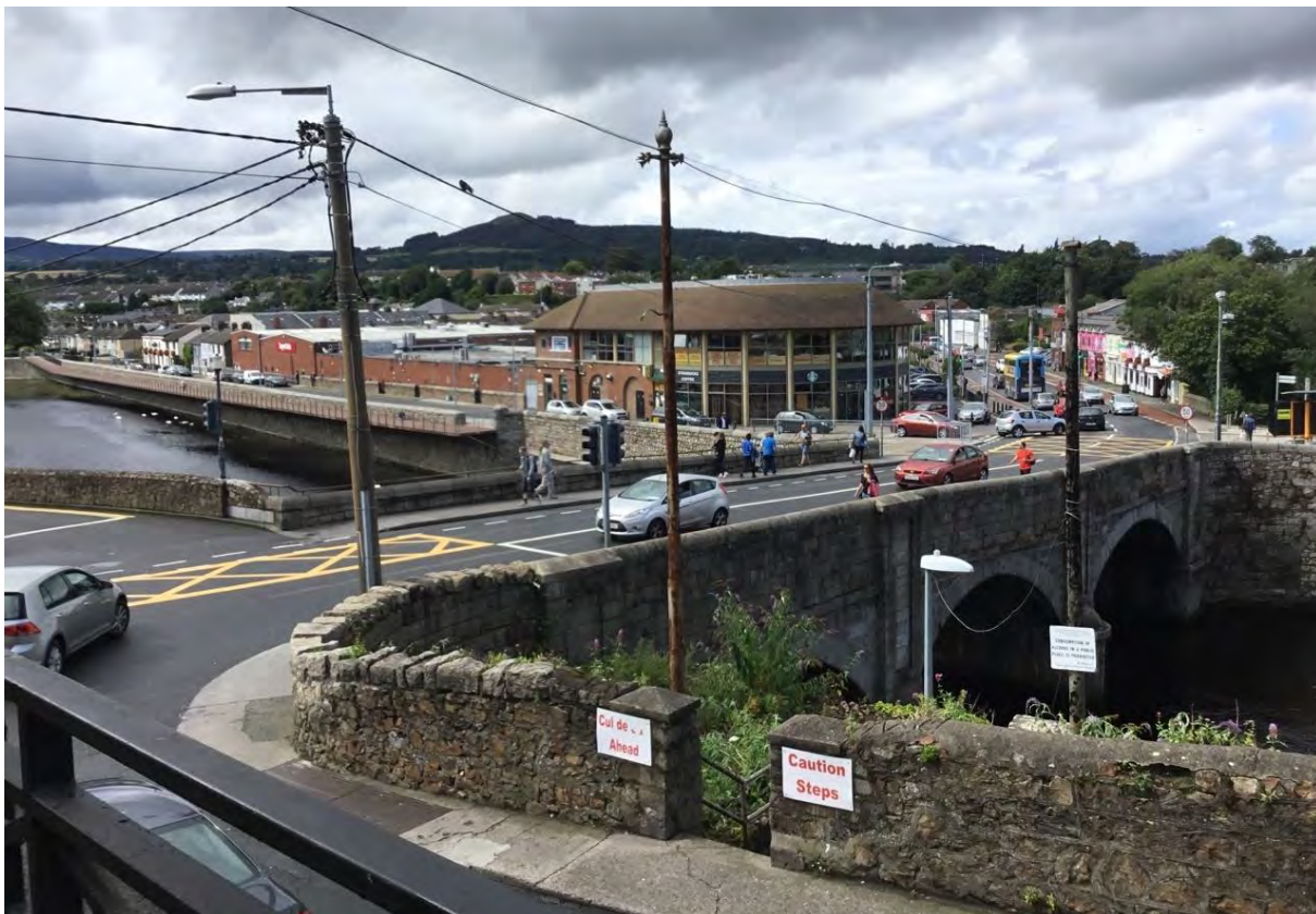
Figure 3.11: View of River Dargle from the south side of the town towards the Super Value store at Castle Street
